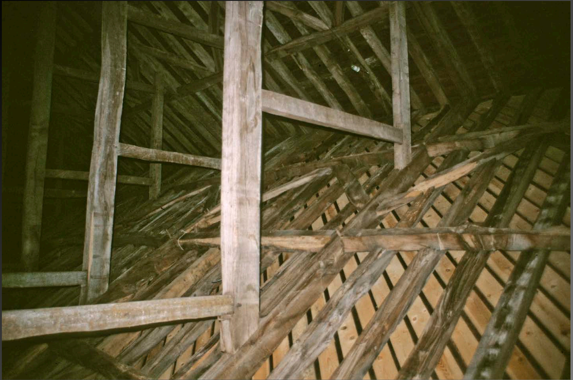
Winchester Cathedral – Roof Void
