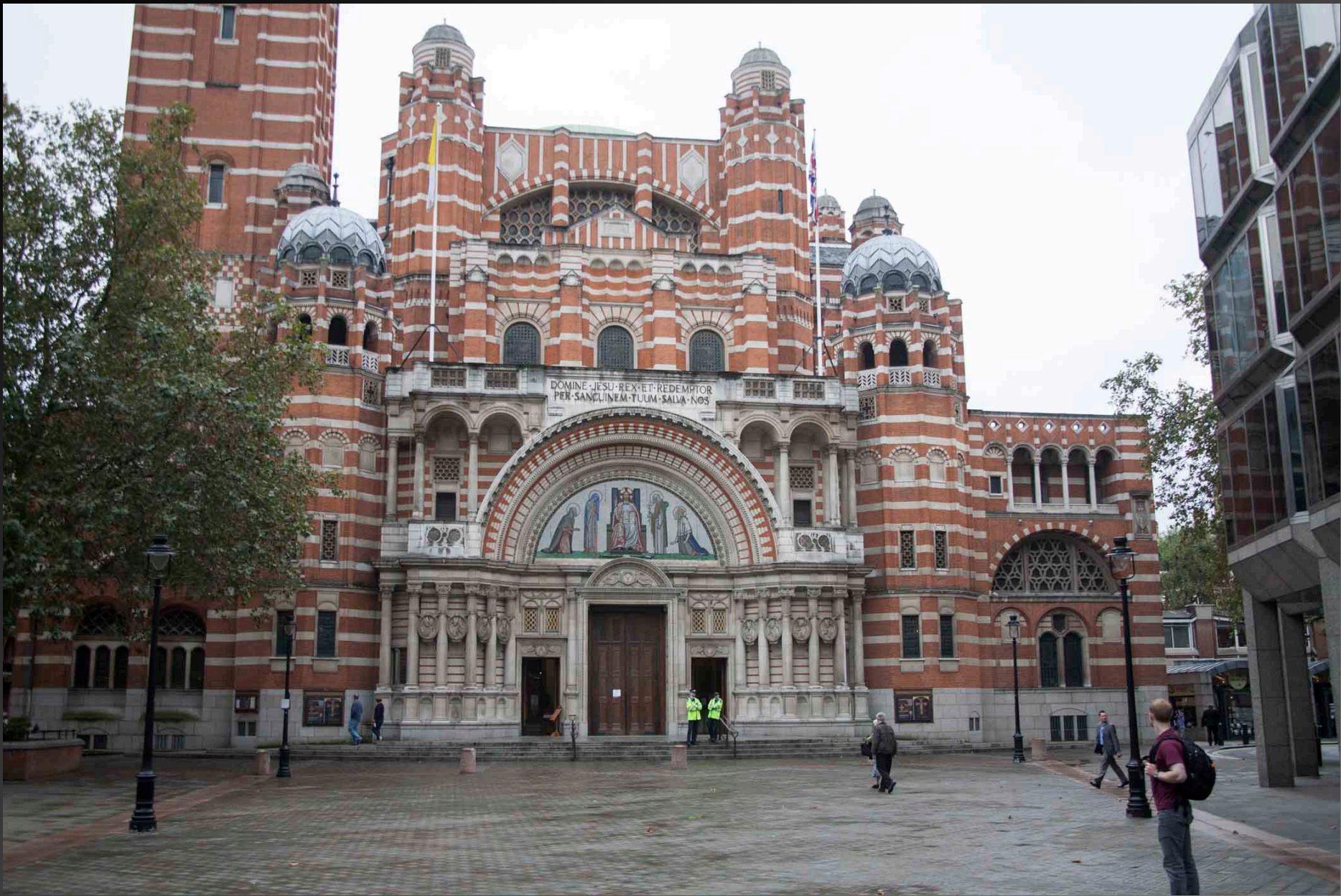
Westminster [RC] Cathedral [still under construction]
